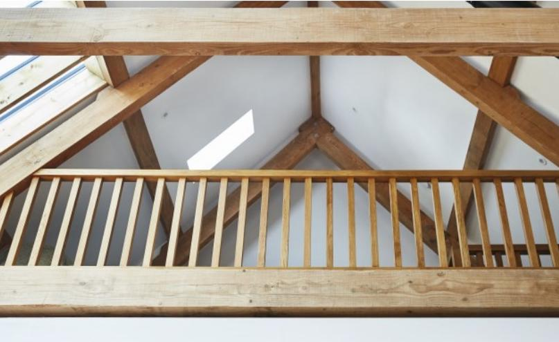
Original beams can be incorporated into the scheme, using steel reinforcement where necessary
